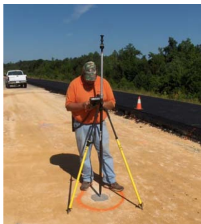
Figure 3.4 Final Survey of Subgrade Earth Pressure Cell
